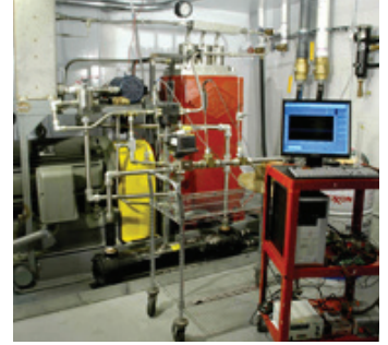
Hydraulic and pneumatic testing
