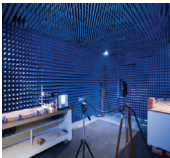
Semi-Anechoic Chamber in Tempe, AZ
