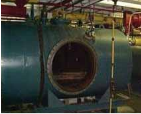
Nuclear steam accident, LOCA, HELB to 600 °F / 300 psig
