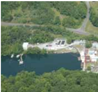
Aerial view of NTS' heavyweight shock test facility, fabrication yard and office complex
